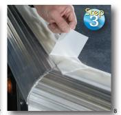
Peel off the release liner.
